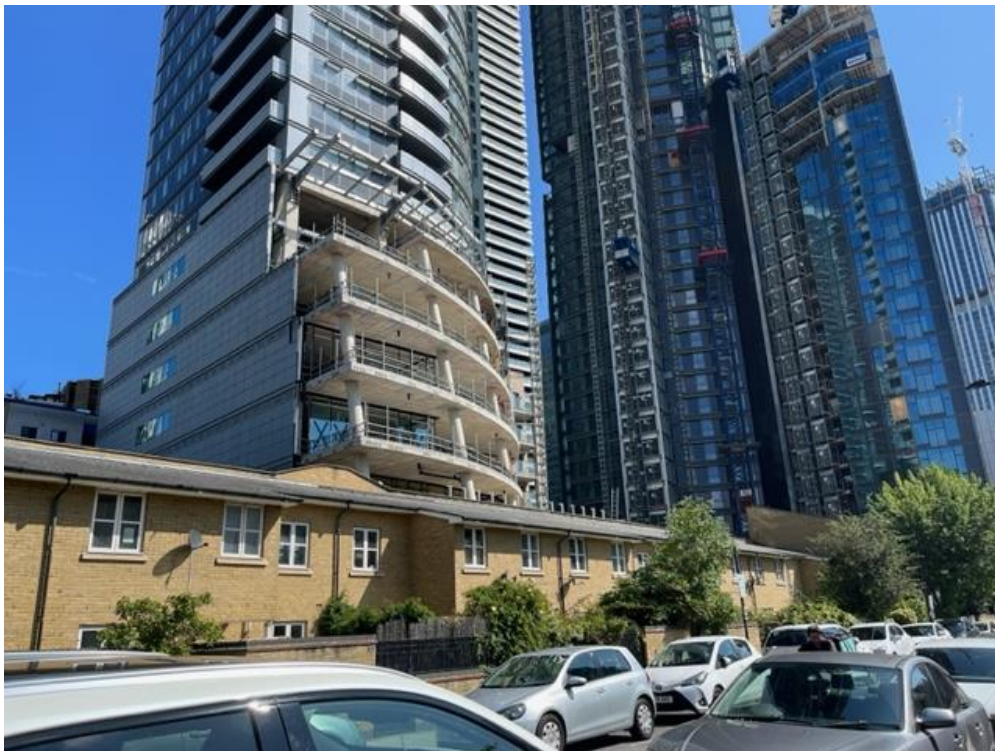
View of Byng Street facing north-west with Alpha Square development behind (taken August 2023).
