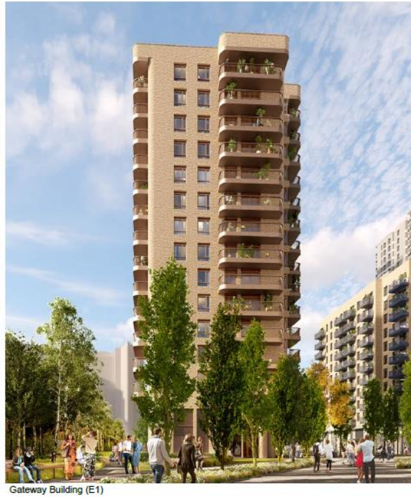
Figure 6 – Architectural treatment of Gateway Buildings.
